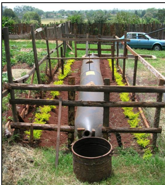
Figure 2-12. Bag digester outside Nairobi, Kenya. The inlet is positioned close to the camera and the outlet in the far (picture from author).
